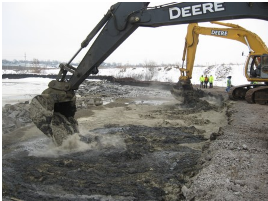
Photograph No. 5 – Mixing Cement
