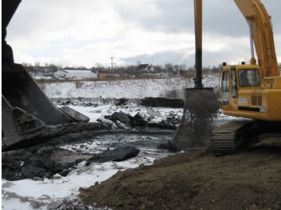
Photograph No. 2 – Slag Addition to Cell
