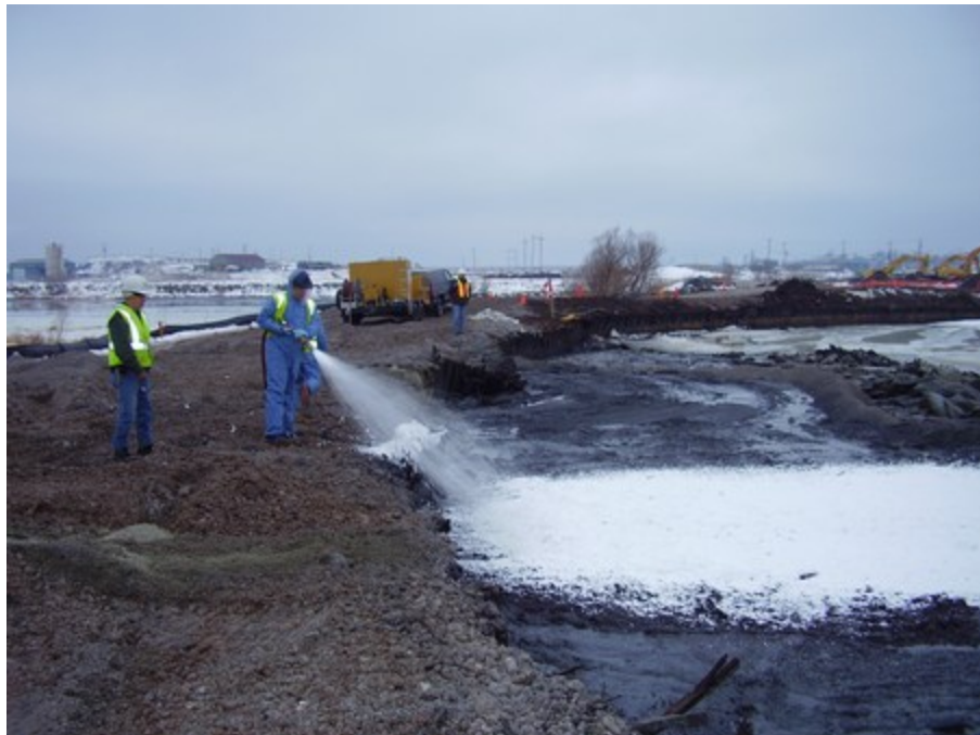
Photograph No. 9 – Foaming after mixing completed
