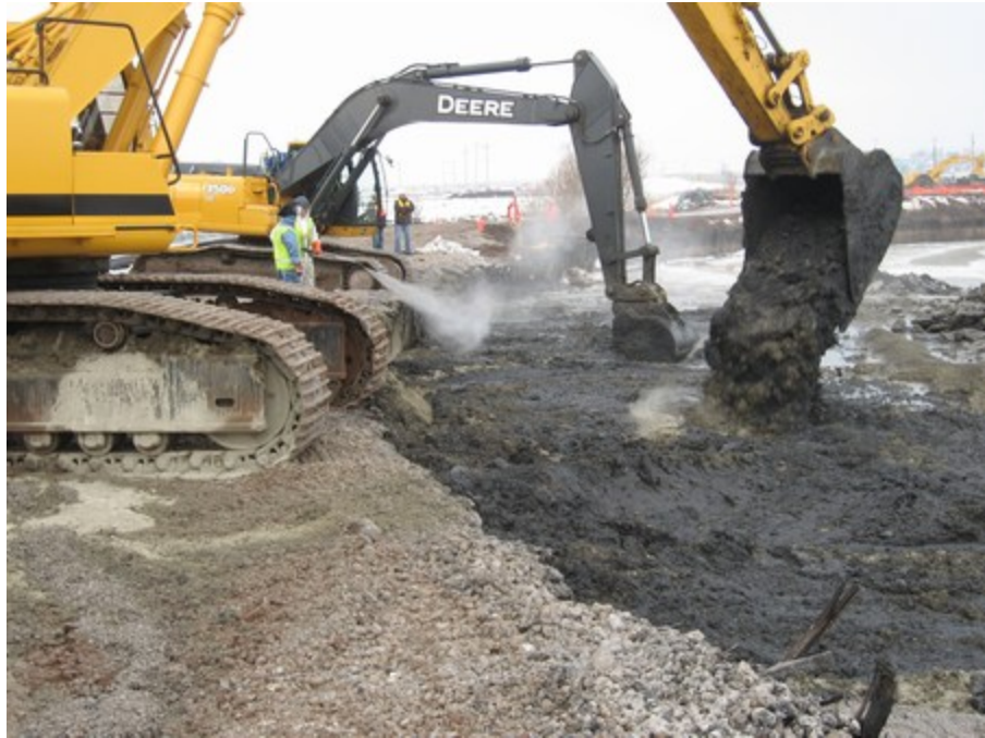
Photograph No. 6 – Dust Control during Cement Mixing
