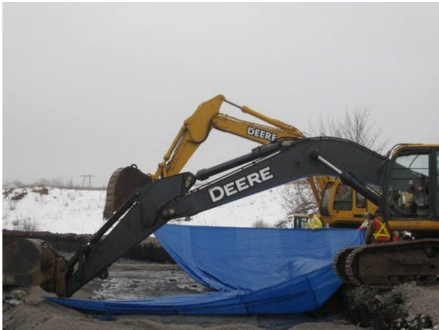
Photograph No. 3 – Tarp Deployment
