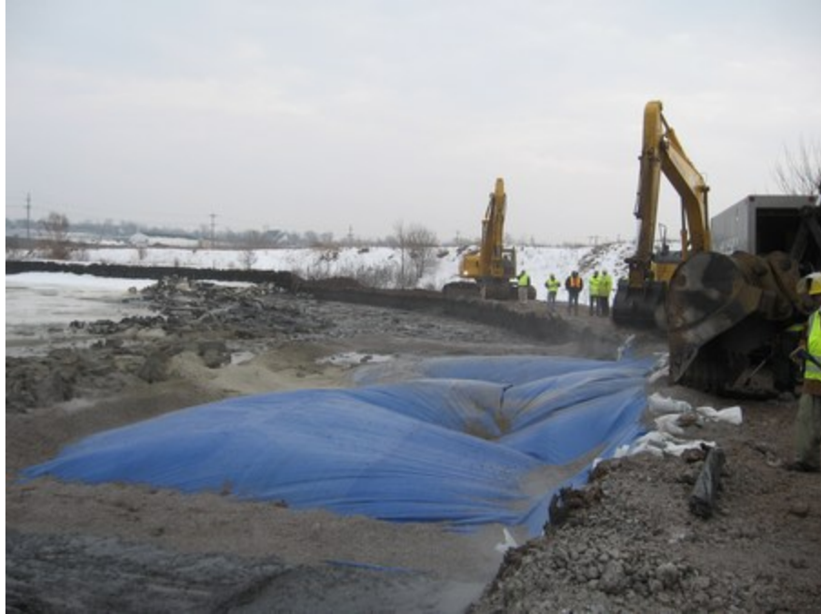
Photograph No. 4 – Cement Addition
