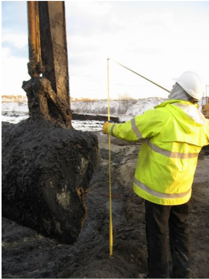
Photograph No. 1 – Measuring Depth of Sediment/Cell
