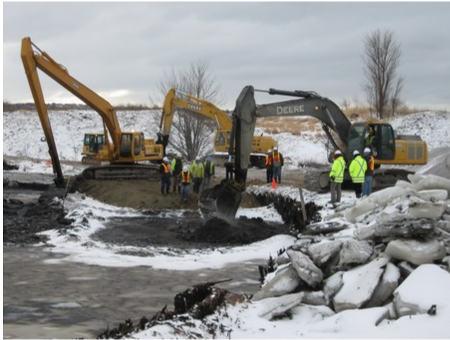
Photograph No. 1 – FD Cell #3 Excavated of Cell After Treatment
