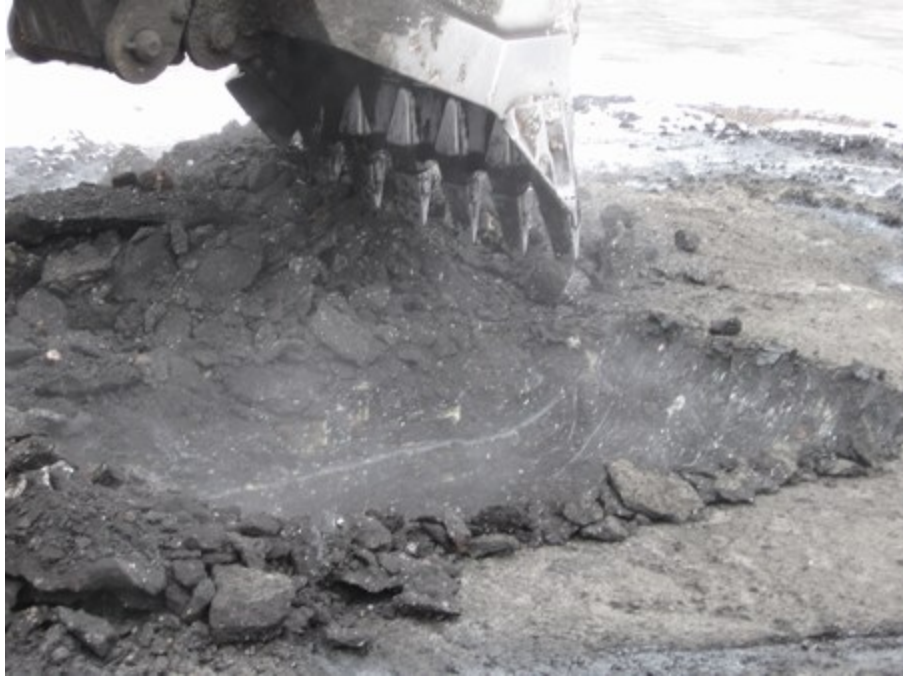
Photograph No. 3 – FD Cell #3 Excavated of Cell After Treatment
