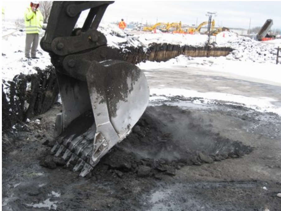
Photograph No. 2 – FD Cell #3 Excavated of Cell After Treatment
