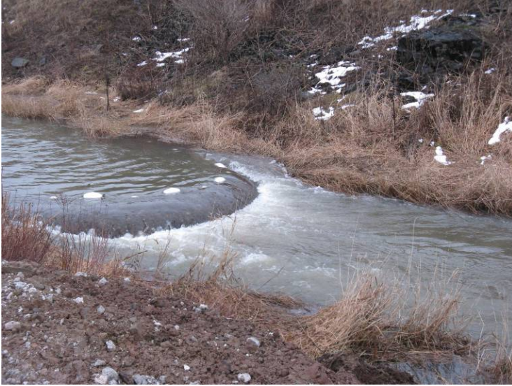
Photo 2 Upper end of Coke Oven Brook closed section showing fish barrier and discharge characteristics.
