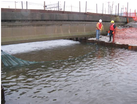
Photo 4 Net placed across Wash Brook.
